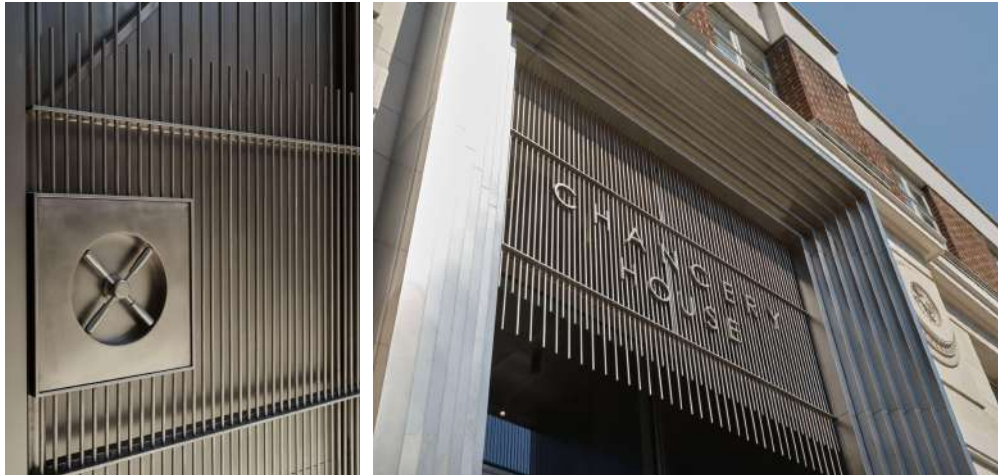
The building's enlarged entrance on Chancery Lane visually references the London Silver Vaults below. Photography by Jake Curtis.
