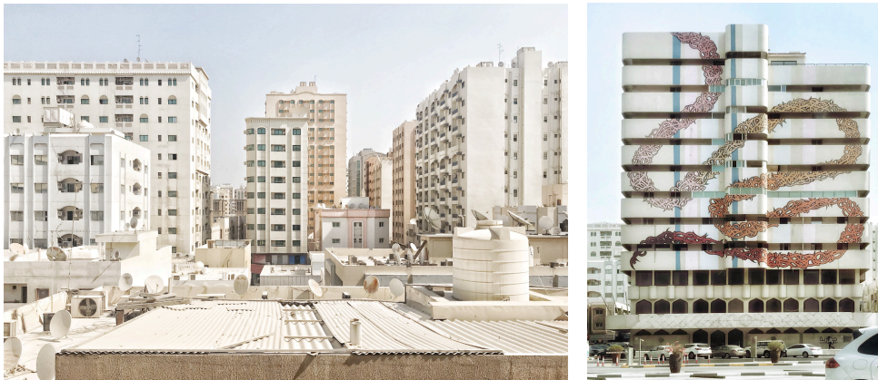
Bank of Sharjah/eLseed Building
