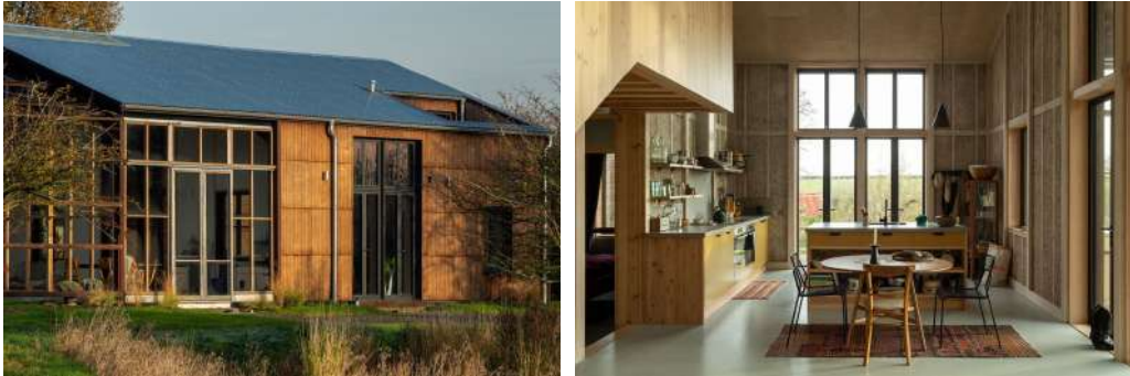
Flat House (2019) at Margent Farm, Cambridgeshire, pioneered the at-scale use of pre-fabricated hemp-based panels in housing construction.
